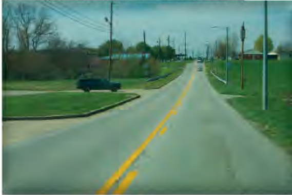
Looking north on KY 658 towards US 68
