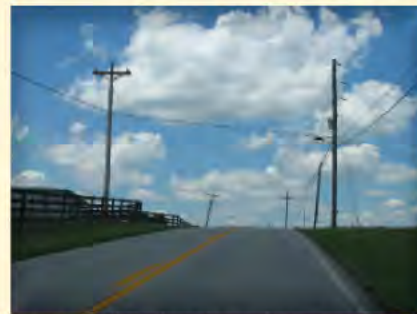
Sight distance deficiencies due to vertical curve approaching an unannounced stop sign
