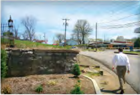
Looking eastbound on KY 70 at the substandard sidewalk
