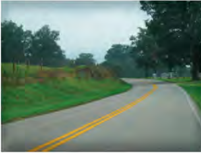
KY 527 Looking north at the embankment and horizontal curve
