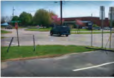
Confusing intersections at MLK Jr. Blvd. and Roberts Road
