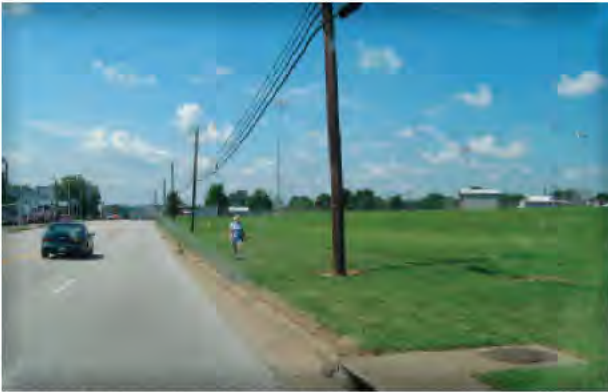
Lack of sidewalks along US 68
